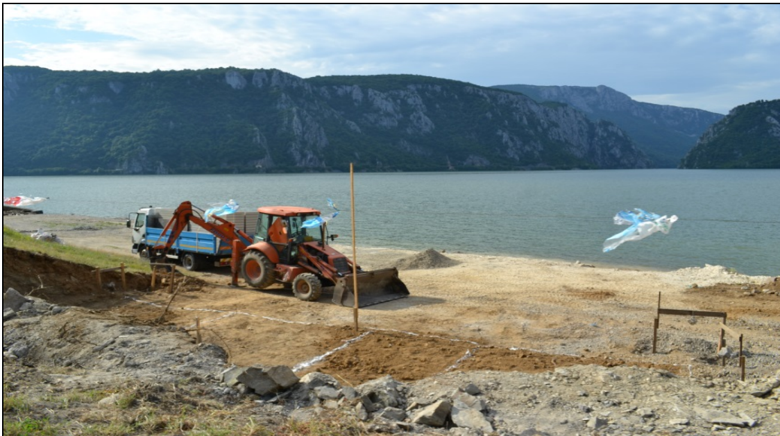
Figure 2: Constructions along the Danube banks at Dubova.
